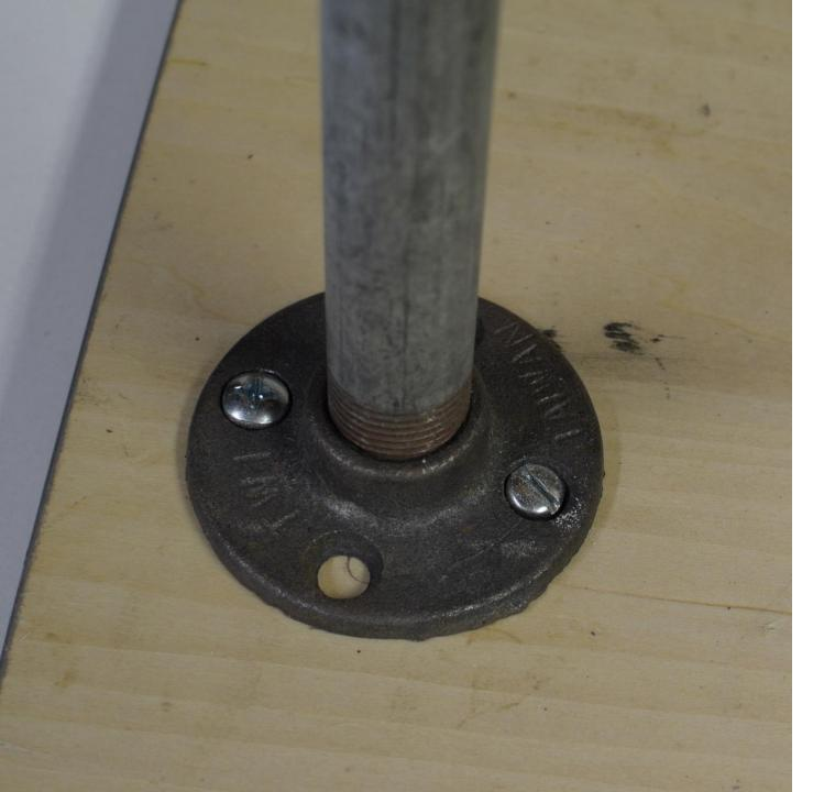
3/4" threaded galvanized pipe Threaded base flange
